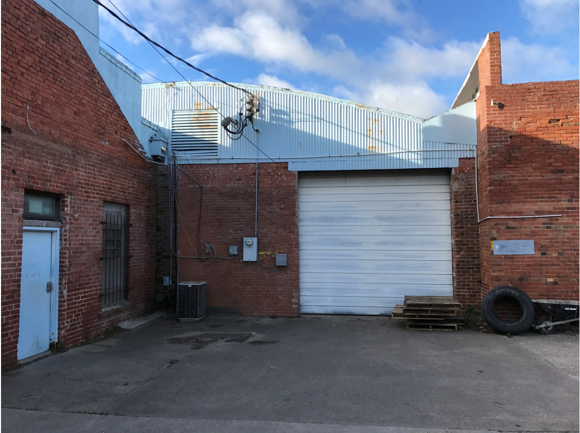
Back View 9 West Broadway
