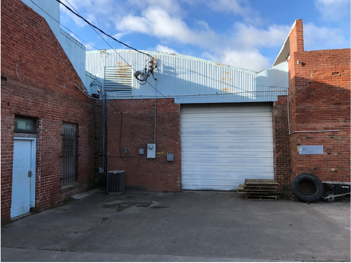
Back View 9 West Broadway
